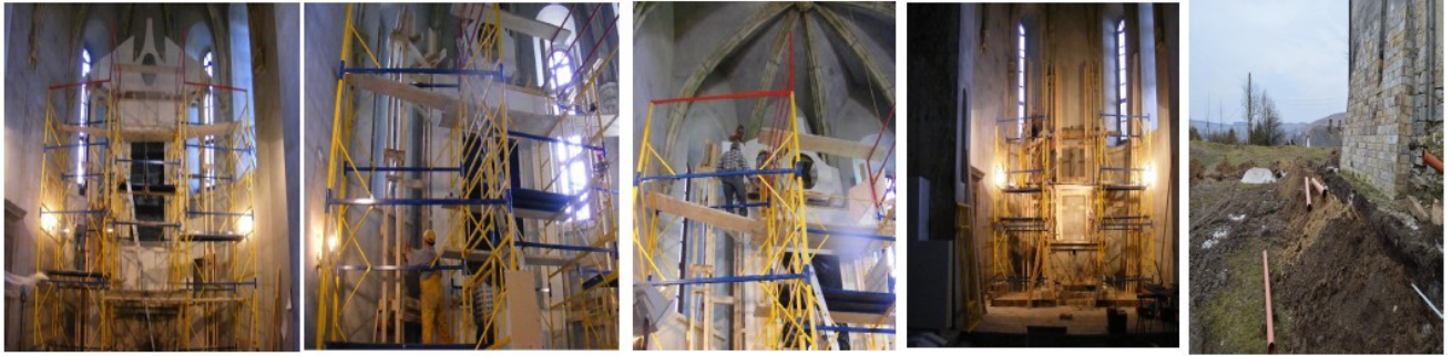
4 PHOTOS OF NEW ALTAR CONSTRUCTION IN PROGRESS
