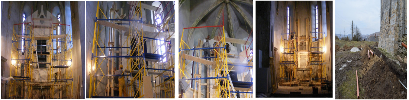
4 PHOTOS OF NEW ALTAR CONSTRUCTION IN PROGRESS
